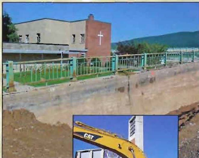
Market St. Bridge Work
