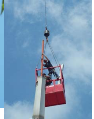
It was then cut in sections at the seams in the aluminum casing, then the steel core.
